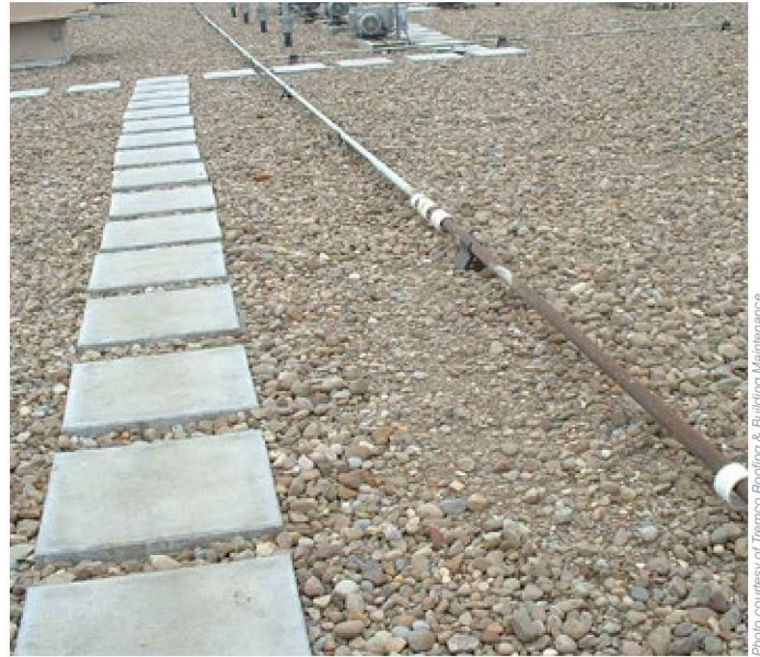
Overview of ballasted roof with concrete pavers acting as a walkway.
