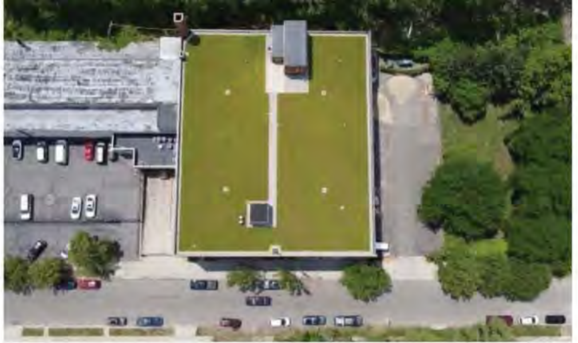
The Belt Line Center building has a 17,250-square-foot extensive green roof and a 2,000-square-foot gravel-ballasted blue roof. A blue roof actually detains stormwater in a rooftop enclosure, in this case, below the gravel-ballasted section. In other cases, the blue roof's enclosure is placed below pedestal pavers or even beneath a green roof's growing media.
