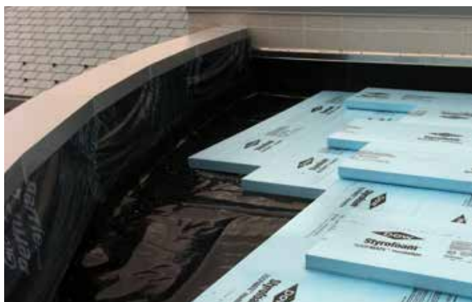
Styrofoam™ Insulation installed
