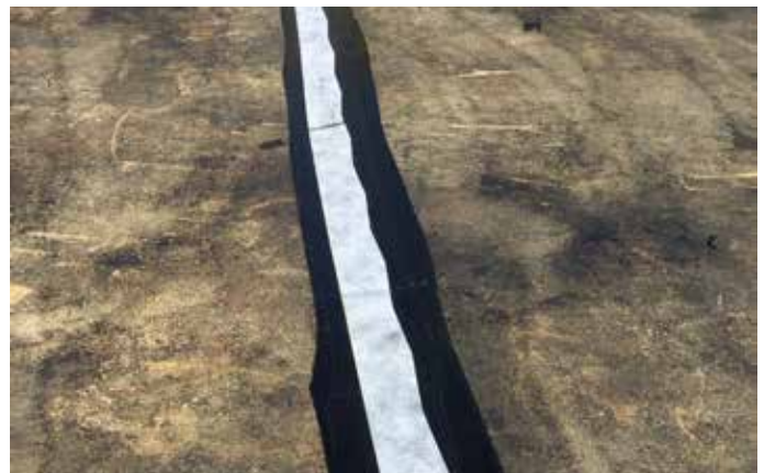
Cold or control joints
