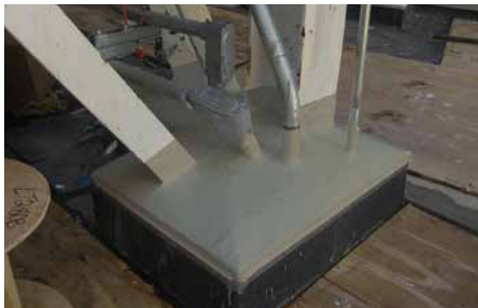
HydroSeal PMMA flashing
