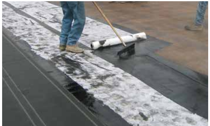
Membrane application in field of deck
