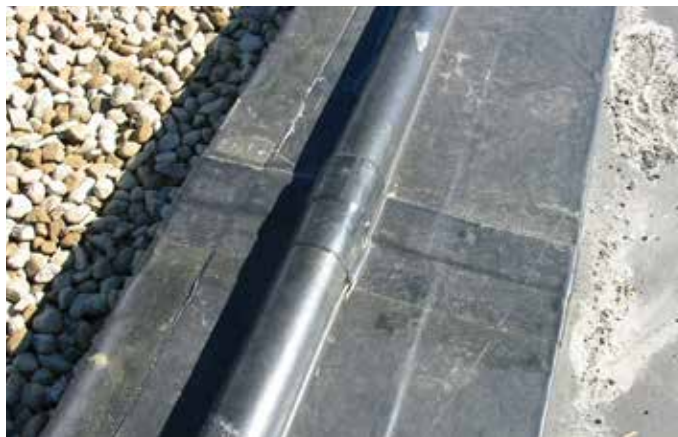
Field fabricated expansion joint
