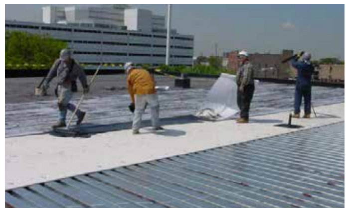
USG Securock Over Metal Deck Substrate
