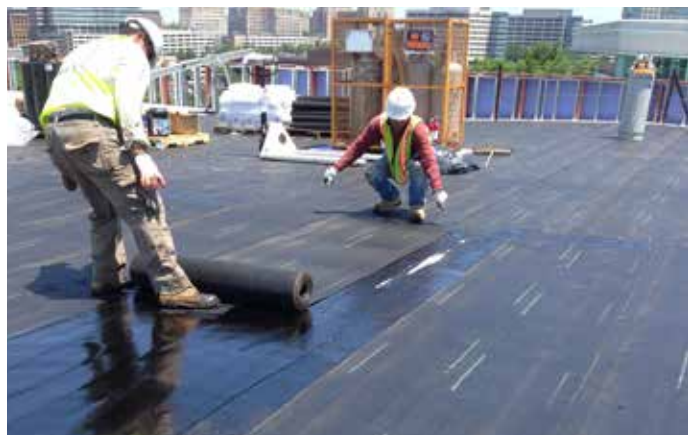
Protection layer installed
