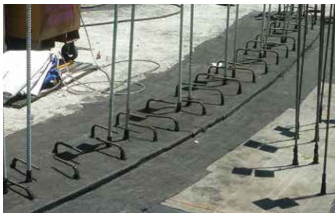
Through wall curb detailing
