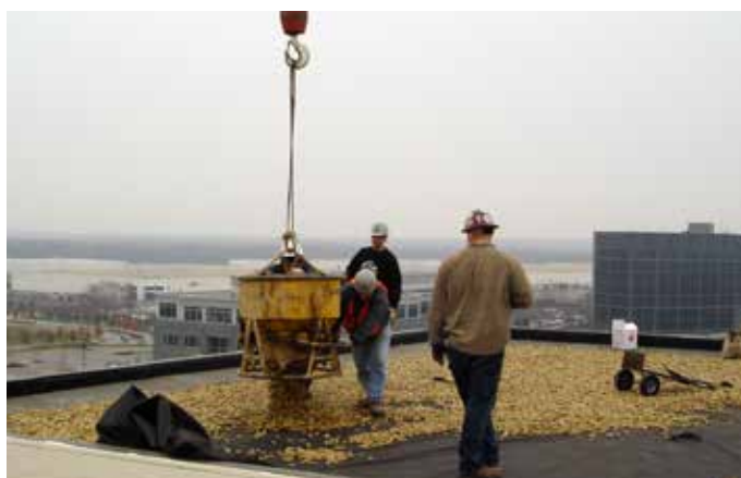
Stone ballast installed
