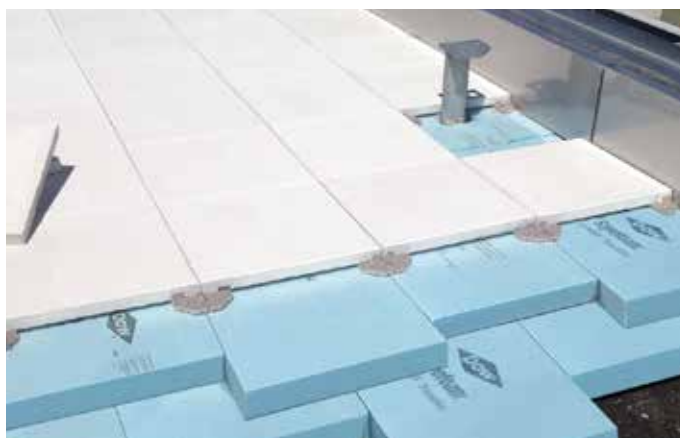
Concrete pavers installed
