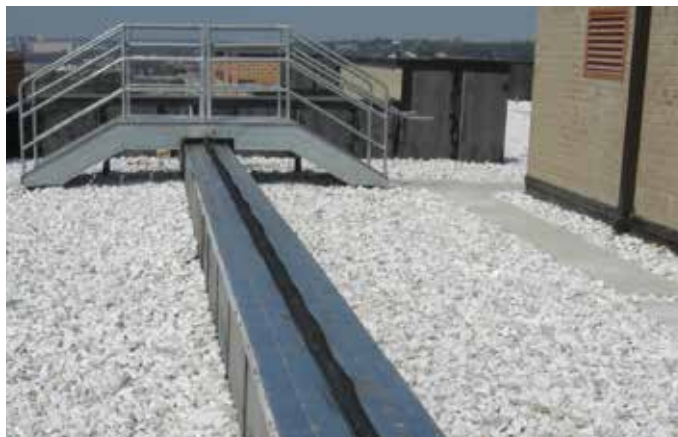
Prefabricated expansion joint
