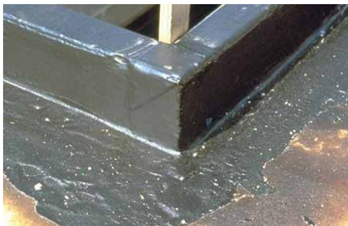
Curb flashing installed
