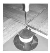
Secure the washer with the screw included. Make sure that washer hooks all four wood tile corners.
