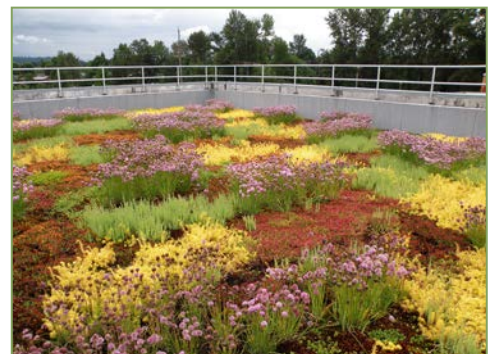
Tri-City Wastewater - Oregon City, OR
