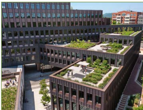
The CODE Building - Charlottesville, VA - Photo: Alan Karchmer
