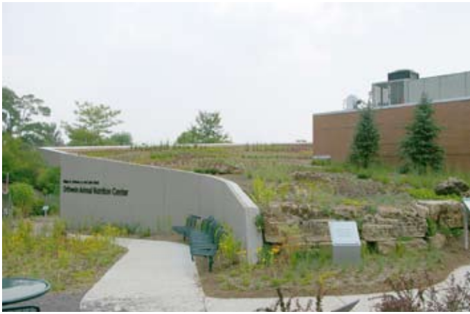
The planting medium, specifically engineered American Hydrotech LiteTop® soil was custom-tailored to provide for optimum infiltration, moisture retention, temperature and insulation, and chemistry for this application of traditional sedums, sedges and Indian grass.
