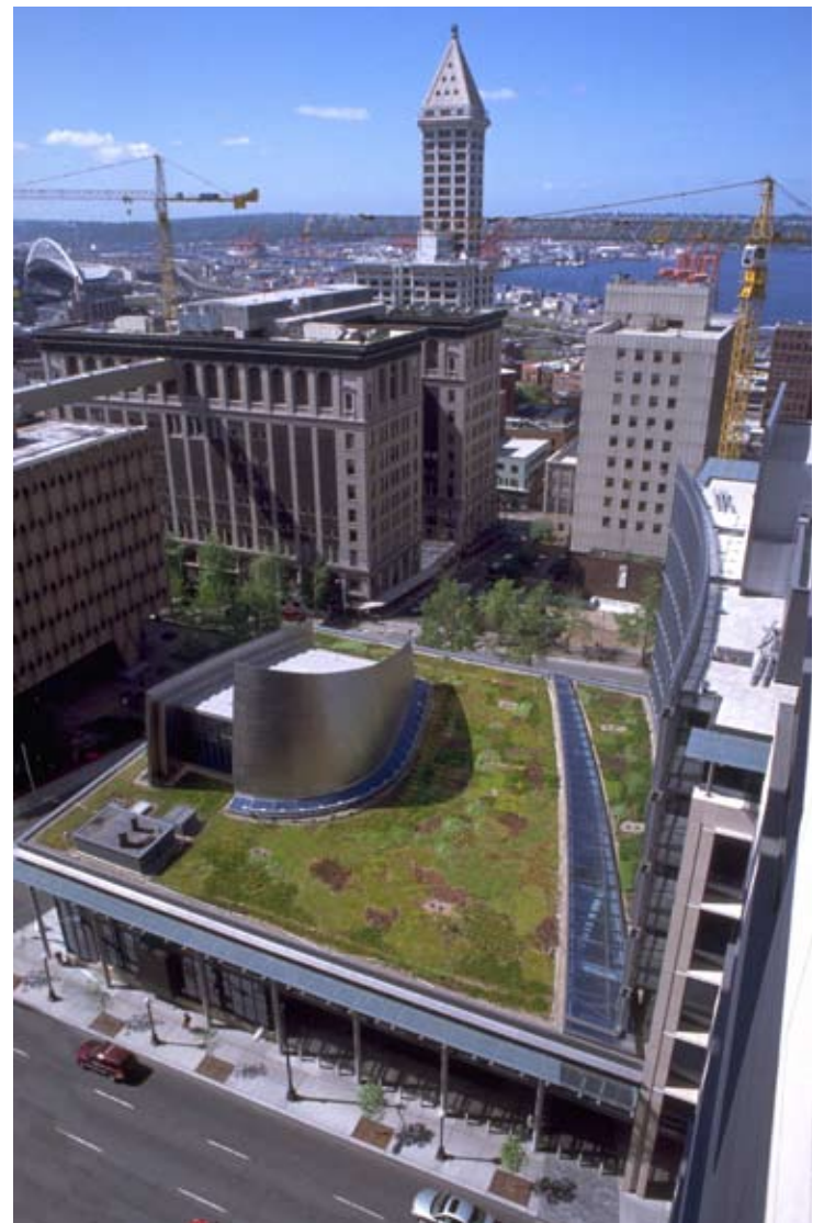
The 13,000 square-foot Seattle City Hall Garden Roof, supplied by American Hydrotech, Inc. Includes a six-inch soil mix and low-growing hardy plants to create a high-profile garden setting that is expected to hold up to the harsh rooftop environment without using a permanent irrigation system.
