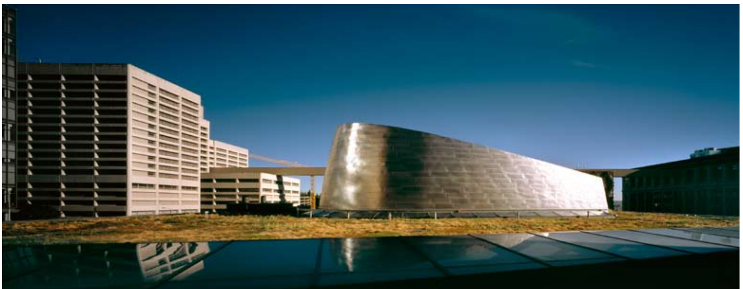
Seattle City Hall's north side is a seven-story office tower, and on the south side of the building is a two-story structure capped with a titanium-clad skylight dome, giving the impression of two separate buildings. The green roofs by American Hydrotech cover portions of both towers, integrating their appearance.
