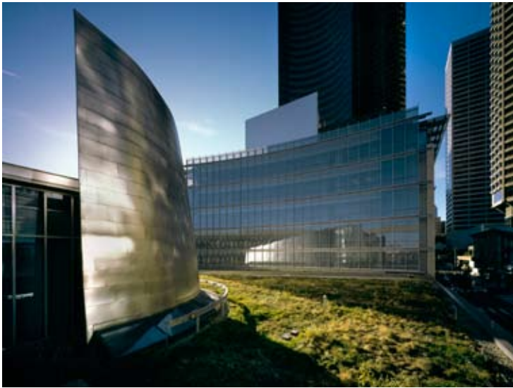
According to Gregory Hepp, principal with Bassetti Architects, who designed the City Hall building through a joint venture with Bohlin Cywinski Jackson, the team chose to do a planted roof as part of their environmental statement and as a LEED® element.
