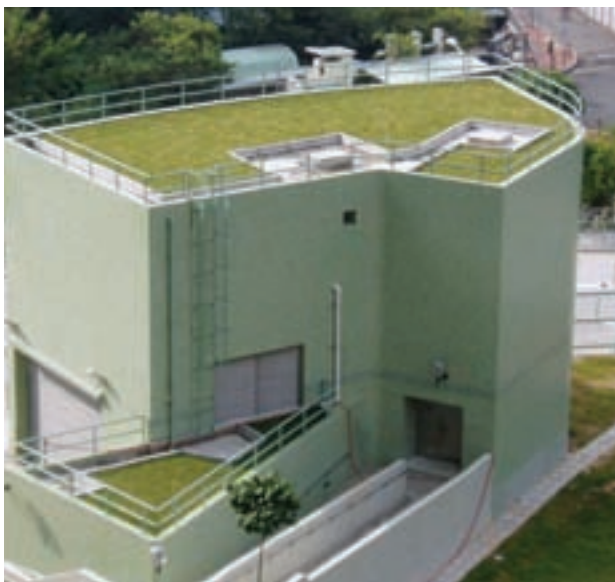
Lei Yue Mun Project, Hong Kong - China
