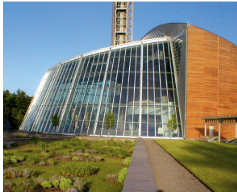
In August 1998, the Mashantucket Pequot Museum and Research Center, Mashantucket, Conn., held its grand-opening ceremony outside the gathering space — on the vegetative roof.
